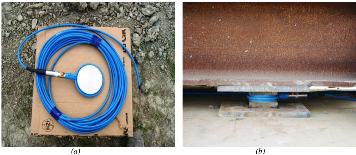
Figure 32: (a) Load cell type Glötzl (b) Load cell installed under steel frame
