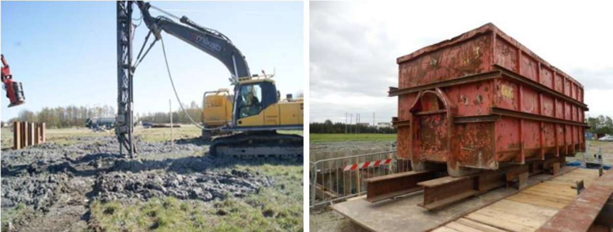
Figure 3: Photo 1: L/C columns and SPW installation; Figure 4: Photo of mounted container in Test 1
