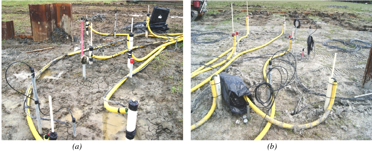
Figure 29: Pictures after completion of instrumentation
