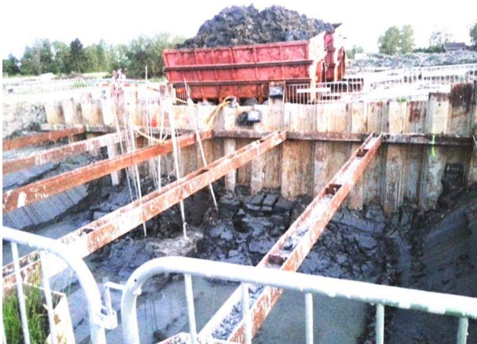
Figure 6: Picture of failure of SPW
