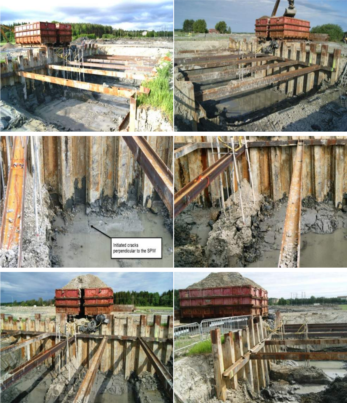
Figure 36: Loading and failure of SPW; Test 2
