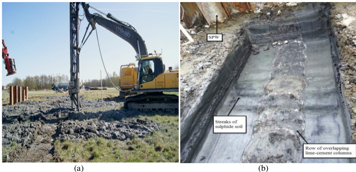
Figure 24: Pictures of Installation of Lime-cement columns
