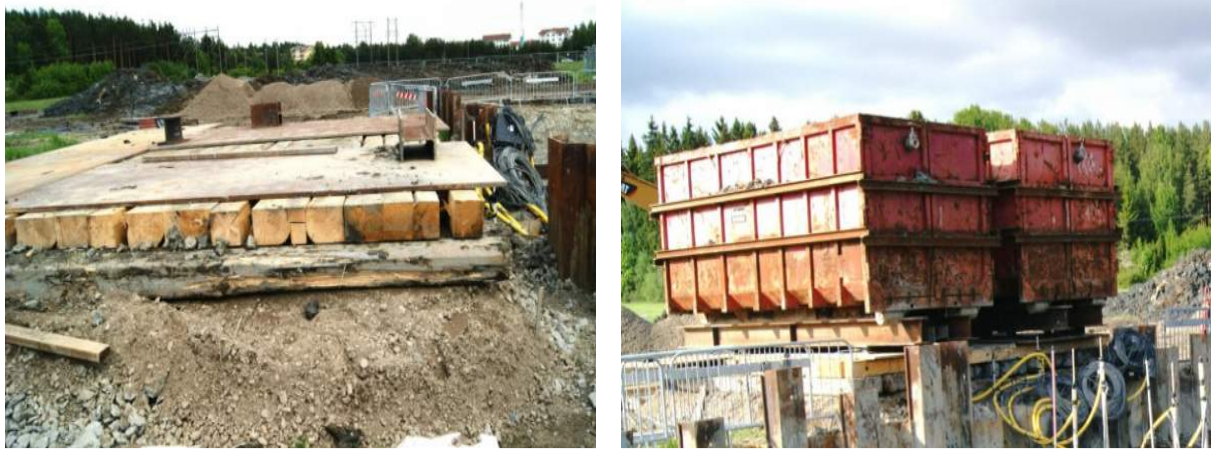
Figure 27: Pictures of LDP construction and mounted container; Test 2
