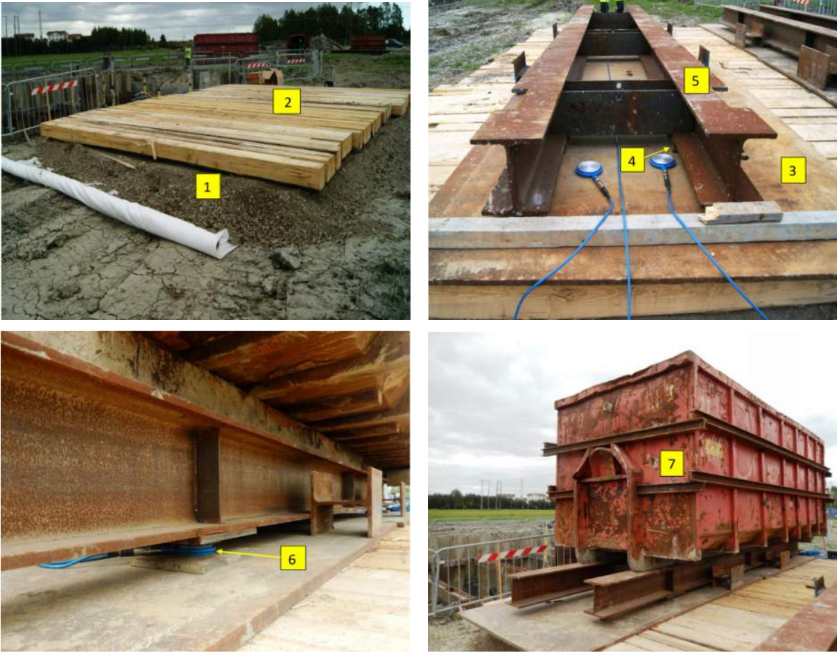
Figure 26: Pictures of LDP construction and load container; Test 1
