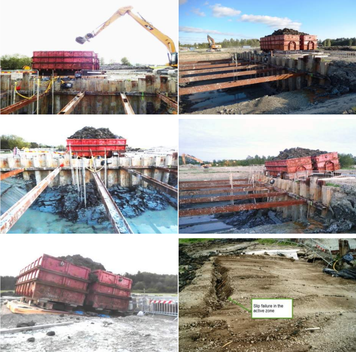
Figure 34: Loading and failure of sheet pile wall Test 1
